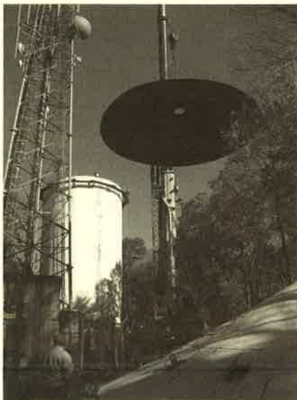
The elder statesman of the Water District's storage facilities has perched atop Great Hill since 1912. The latest inspection showed the riveted-steel Great Hill tank to be in good shape, but in need of a new "cap". The integrity of storage tanks is critical, so a brand new custom "hat" was designed for the tank. It took a sixty-ton crane and crew of several engineers to hoist and weld the new cap in place, giving it a jaunty, more modern look.
