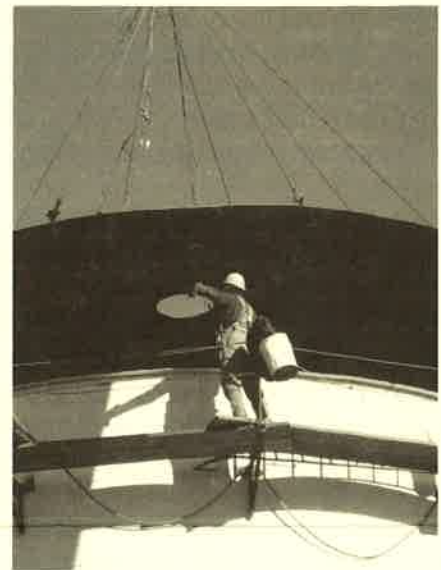
The elder statesman of the Water District's storage facilities has perched atop Great Hill since 1912. The latest inspection showed the riveted-steel Great Hill tank to be in good shape, but in need of a new "cap". The integrity of storage tanks is critical, so a brand new custom "hat" was designed for the tank. It took a sixty-ton crane and crew of several engineers to hoist and weld the new cap in place, giving it a jaunty, more modern look.
