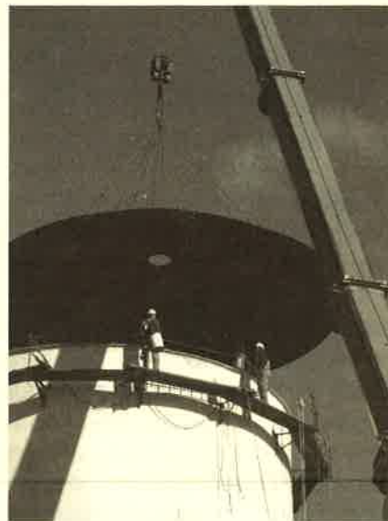
The elder statesman of the Water District's storage facilities has perched atop Great Hill since 1912. The latest inspection showed the riveted-steel Great Hill tank to be in good shape, but in need of a new "cap". The integrity of storage tanks is critical, so a brand new custom "hat" was designed for the tank. It took a sixty-ton crane and crew of several engineers to hoist and weld the new cap in place, giving it a jaunty, more modern look.
