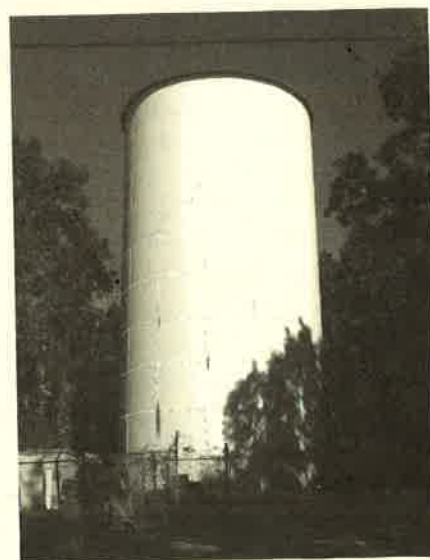
Storage of water, in above-ground tanks like this standpipe at Great Hill, can provide water in times of power outages.
